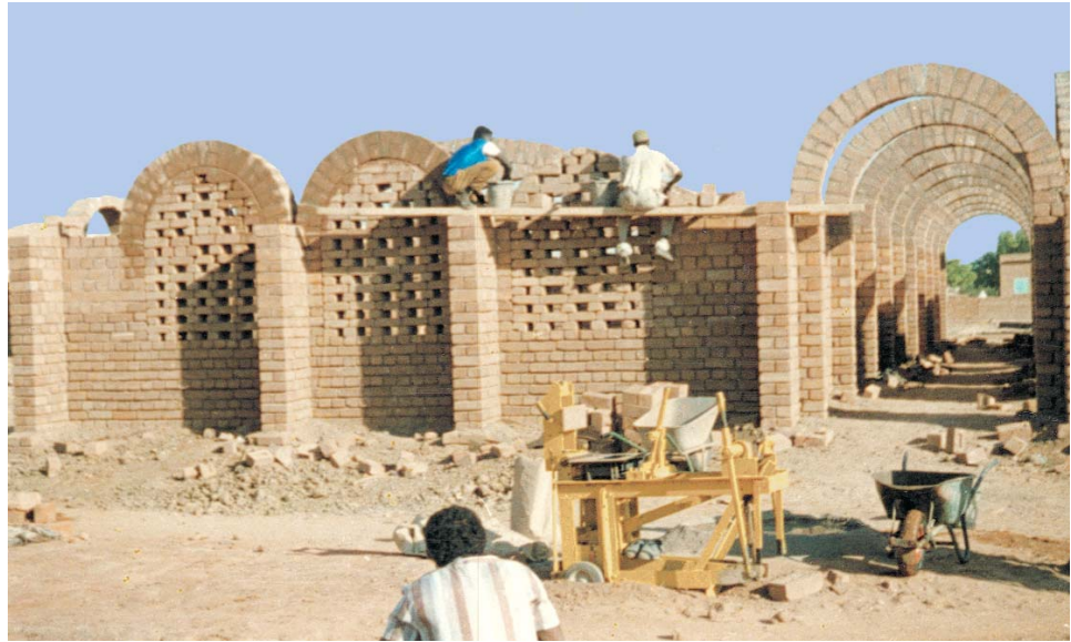
Figure 7.1 - El Haj Yousif school under construction
